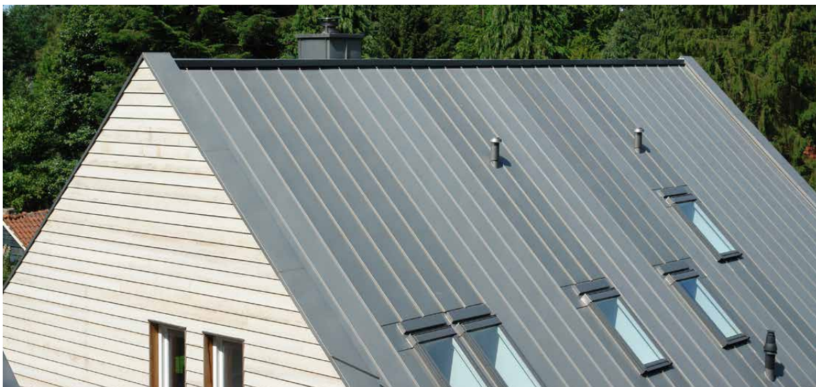
Colour differences on a pitched roof
