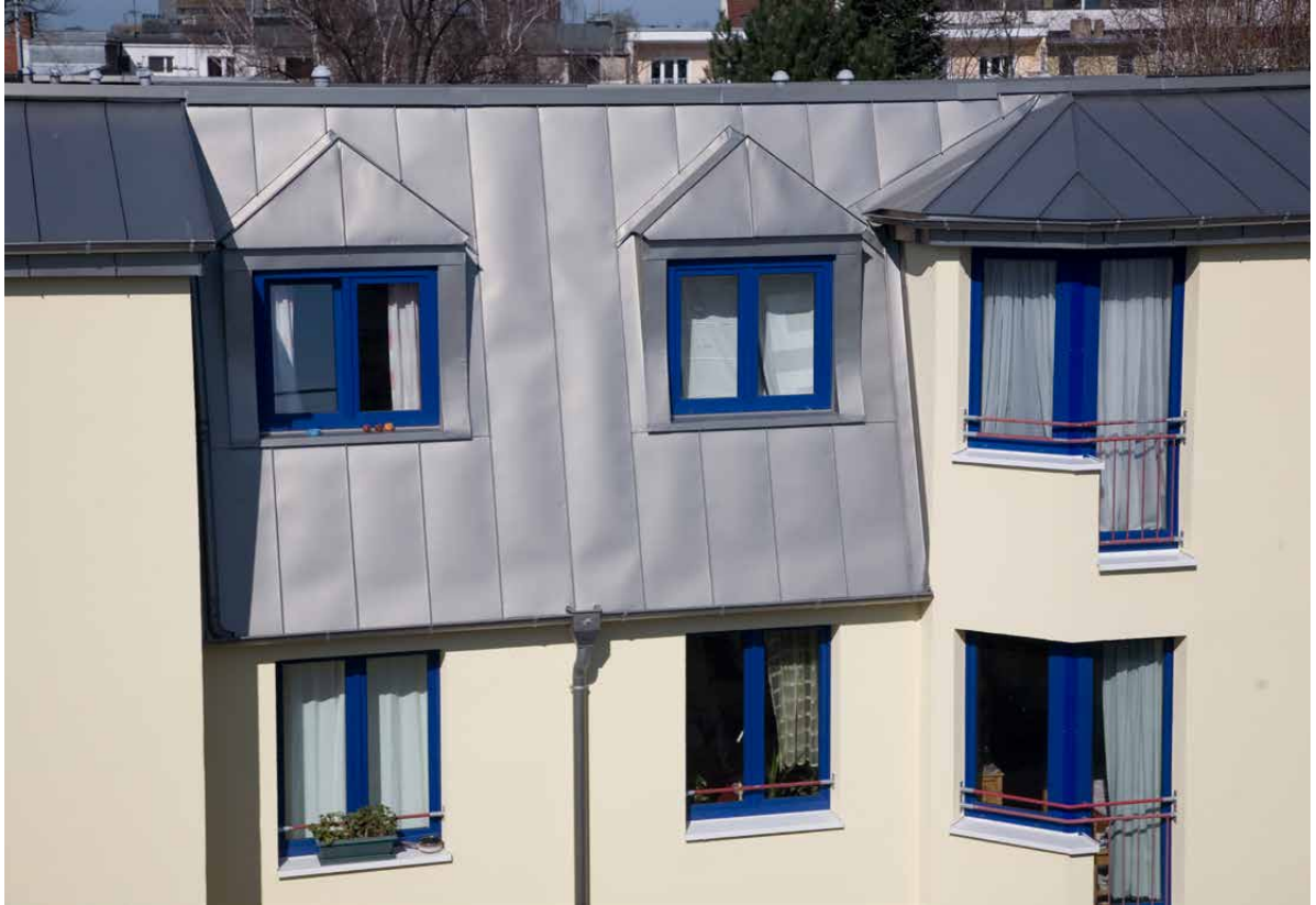
Visible oil canning on a sunny day
